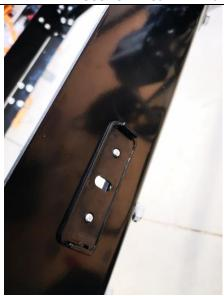
The wires get fed through the hole in the bracket and then the light snaps into place onto the bracket
